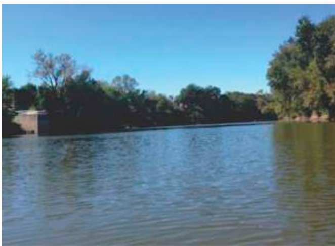
Defiance has a vested interest in water quality across the Maumee watershed; the River serves as our primary drinking water supply and provides recreational opportunities to the community.
